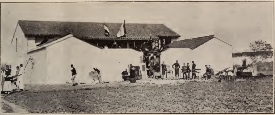
A typical Chinese church building.
